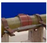
A special interior heating collar is used for flange joints 3" and smaller. Make sure that contact is made between the heating collar and pipe wall. Heat for the recommended time.
