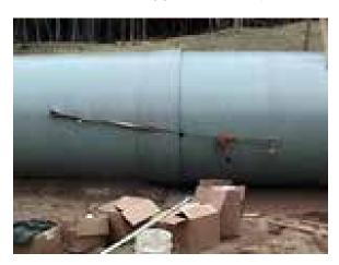
b) Joining force can be applied with come-a-longs and cables, attached between lugs, provided for that purpose. Do not push joint together with excavating machinery.
