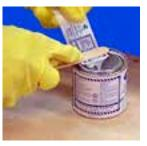
NOTE: The P1500 and H1500 catalyst pillow pouch contains ingredients that tend to separate after a short time. To ensure all of the ingredients are added to the adhesive, mix the contents by hand prior to opening the pouch. Gently mix by squeezing with your fingers until the two (2) catalysts are well mixed. Be careful not to apply excessive pressure, as this may result in damage to the pouch.
