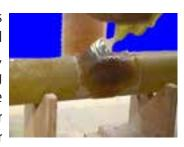
all overlapped ends are staggered around the joint. NEVER ALLOW THE GLASS TO SAG.
