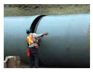
e) Align the pipes in line with each other within  $\pm 11/2^{\circ}$ .
