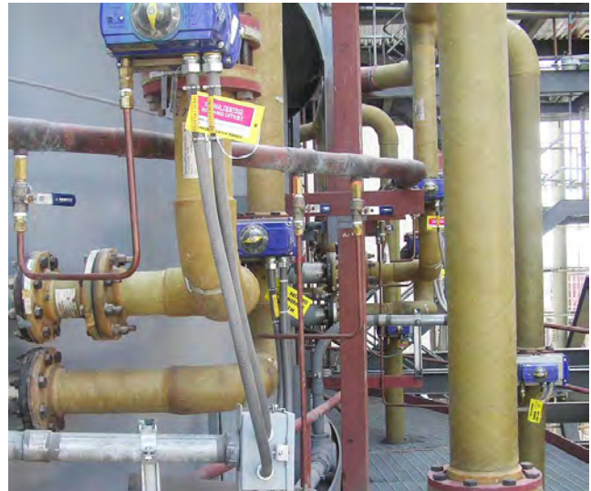
HPPE P-150 in service at a chemical processing plant.
