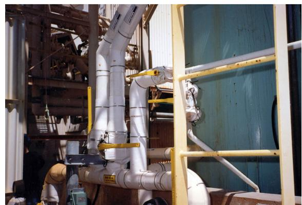
Minimally flanged installation for sulphuric acid in service since 1996.
