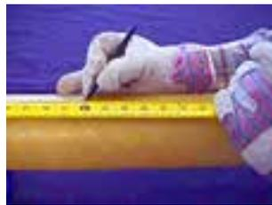
Pipe end must be square to within tolerance (face to center-line dimension  $\pm 1/8"$  up to and including 12" dia., or  $\pm 3/16"$  for 14" dia. and larger).
