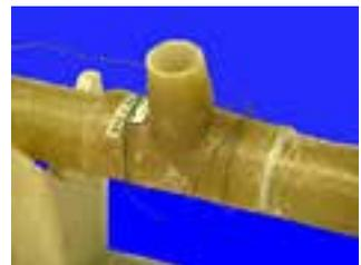
i) Apply two (2) heating collars **longitudinally to each side** of pipe saddle for 105 minutes.
