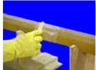
g) Using a mixing stick - smooth out excess adhesive forming a neat fillet at the edges of the saddle, and remove any adhesive that may block the hole in the pipe.
