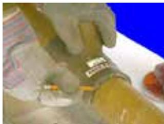
c) Remove PEEL-A-BOND™ material from pipe saddle. Refer to RPS Pipe and Fittings Installation Manual, Page 51.
