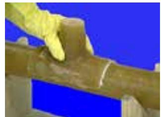
h) Apply two (2) heating collars; one (1) to **each side** of pipe saddle for 105 minutes. Do not attempt to combine steps h) and i), as overlapping may damage a heating collar thermostat and lead to an uncured or overheated joint.
