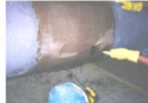
GET THE REINFORCEMENT - WET OUT THE REINFORCEMENT - APPLY THE REINFORCEMENT - ROLL OUT THE REINFORCEMENT
