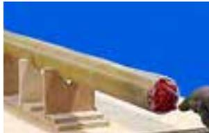
Do not pull the Pig through the pipe until the joint has been secured.
