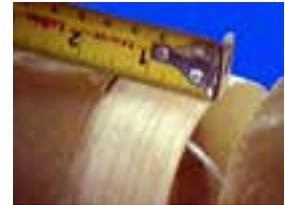
**NOTE:** In fitting to fitting joints, the fitting ends must not touch. If ends touch, the fit must be corrected to the correct gap as per fitting dimension sheets (see RPS Dimensions Catalogue for dimensions).
