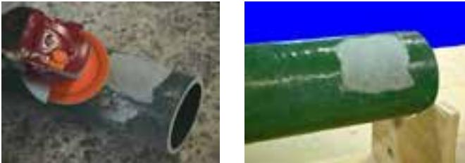
Remove all loose dirt and dust with a rag or a blast of dry, oil-free air.
