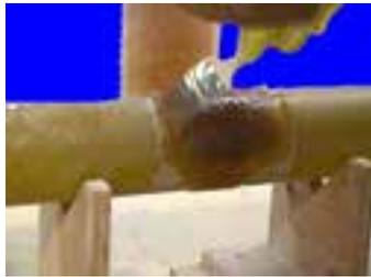
After each step of reinforcement (5 layers) is applied, the lay-up must be allowed to cure for 30 minutes to 2 hours depending on the temperature and the amount of catalyst added. During cure, the lay-up generates a considerable amount of heat. Do not commence the next step until the lay-up has cooled (you should be able to hold your hand comfortably on the laminate).
