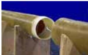
Insert the Pig into the pipe on one side of the joint, and thread the rope through the pipe on the other side.
